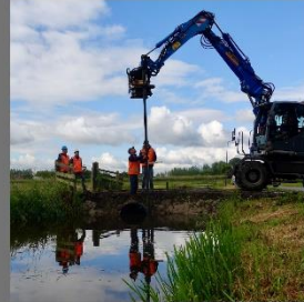
Poles to mark culvert
