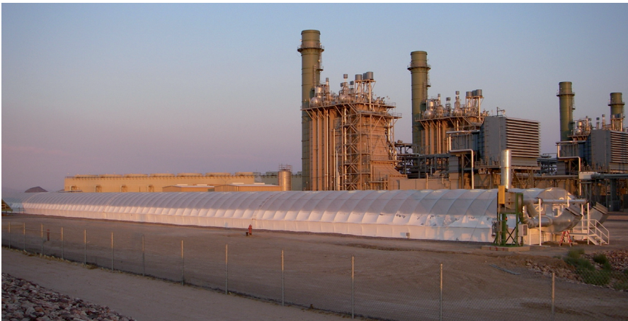
Abbildung 6: APS Red Hawk Power Plant, Phoenix, Arizona
