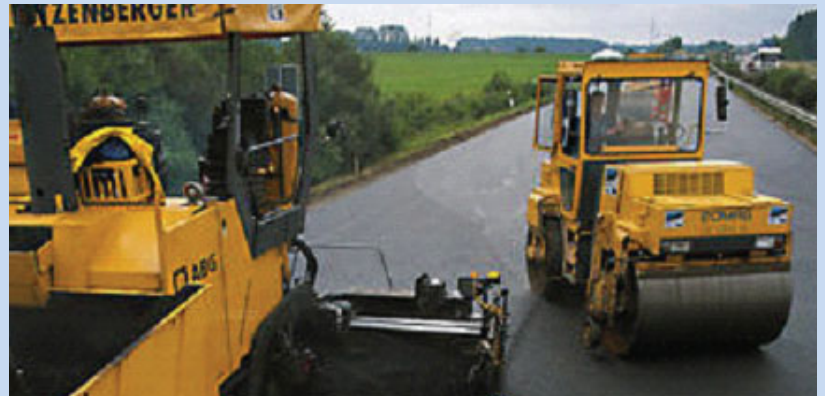
Right: Bottom ashes, leftover from biogenic waste incineration, are commonly treated and reused in construction projects like road paving in Europe.
